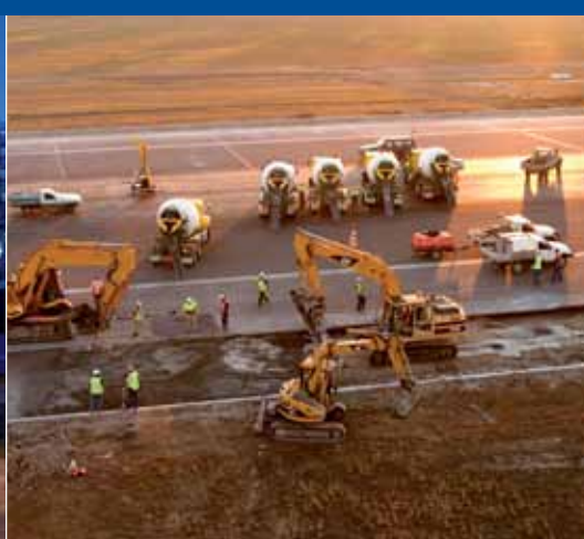
Melbourne Airport A380 Runway Widening
